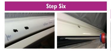
Apply a tiny amount of the sealant over each pre-drilled hole in the van. With the help of an assistant, hold the rail in position being very careful not to smudge the sealant bead. Fix the rail into the pre-drilled holes with your PH2 hand screwdriver using the supplied chemically blacked stainless steal screws. Again, start from the middle, work towards the front, and then from the middle towards the rear. TAKE CARE-NOT TO OVERTIGHTEN THE SCREWS the sealant is the main fixing once cured.
